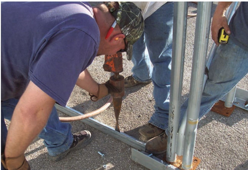
ANCHOR BASE RAIL TO THE SURFACE AREA
