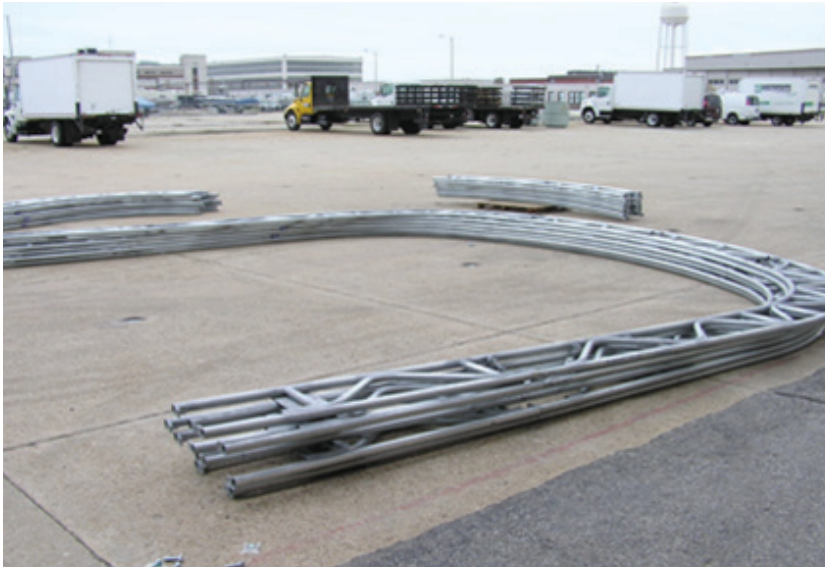
ASSEMBLE TRUSS FRAMES
