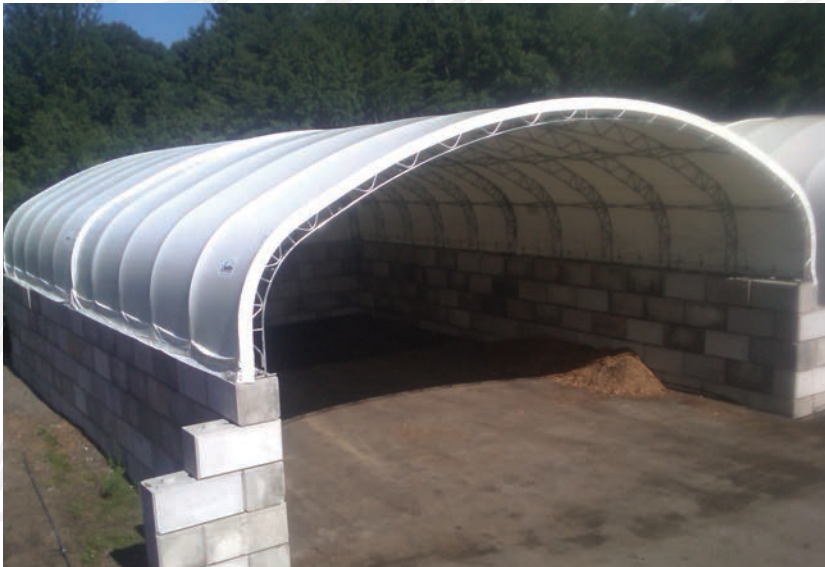
INCREASE STRUCTURE'S HEIGHT/SIDEWALL CLEARANCE
