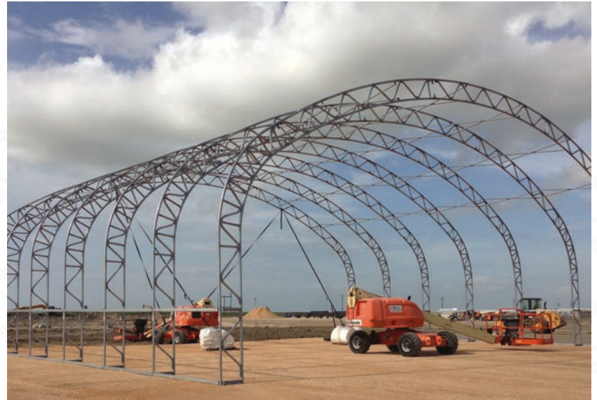
STAND TRUSS/INSTALL X BRACES & PURLINS
